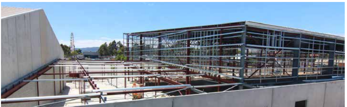
State Basketball Centre development, photo care of Pike Construction
